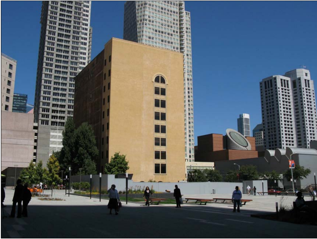
(E) VIEW OF PROJECT SITE FROM WEST
